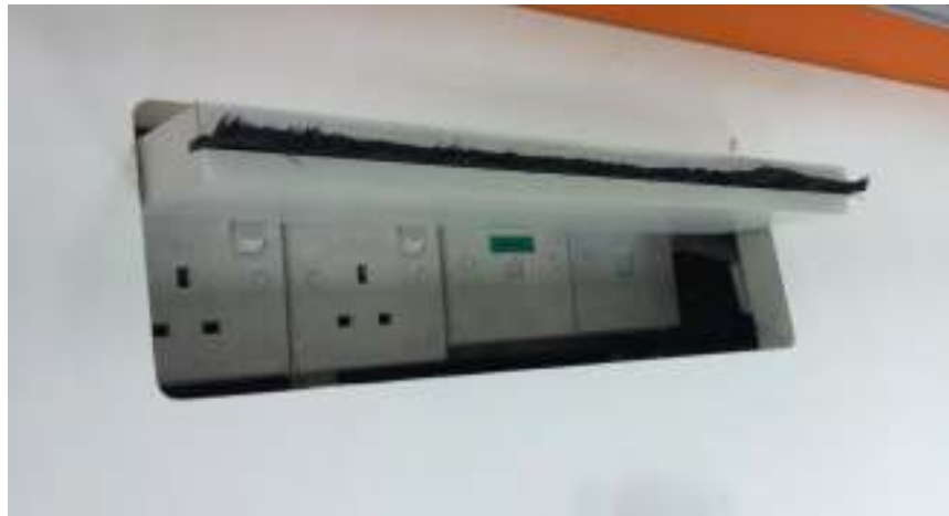
Flipper Cover + Bottom Wooden Box ( for wire socket )
